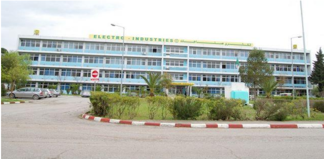
Figure 1: Infrastructure de l'entreprise ELECTRO-INDUSTRIES.
