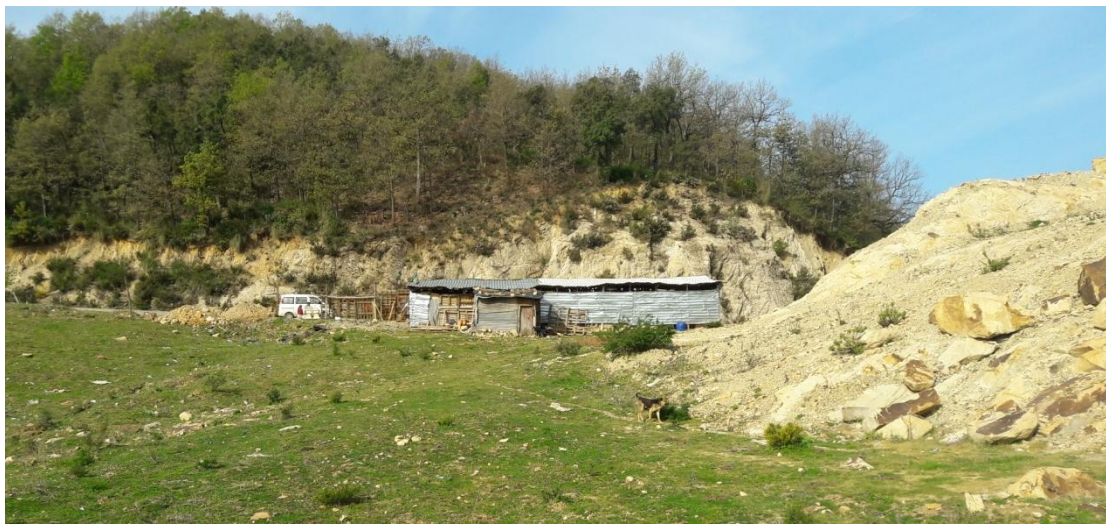
Figure 32. Installation de commerces illicites (coté Est).
