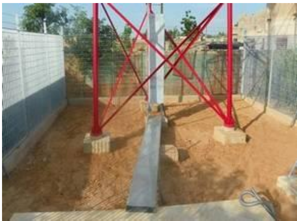
Figure II.9: Installation du Pylone.
