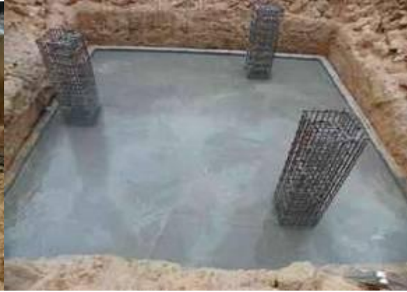
Figure II.8: Plateforme du Pylone.
