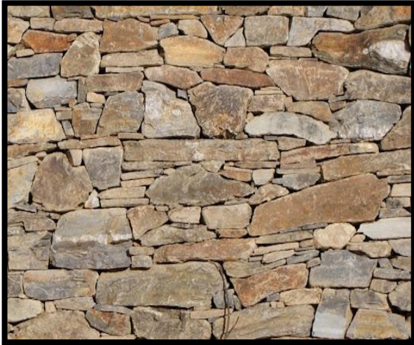
Figure 138: Pierre de construction source google image
