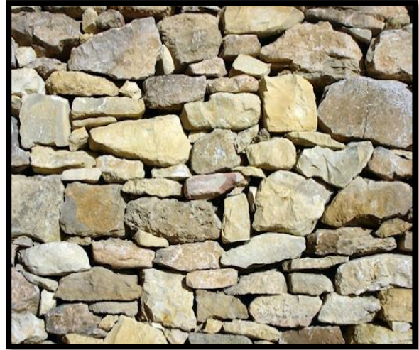
Figure 137: Pierre de construction source google image
