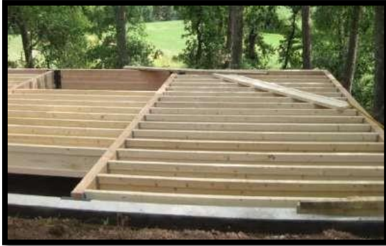
Figure 154: pose de bois Source : https://www.pinterest.fr/homefeed/
