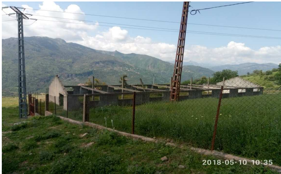
Figure 3 : Site de compostage.
