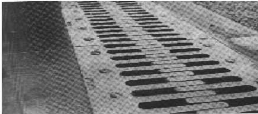
Figure XV-4: Joint de chaussée
