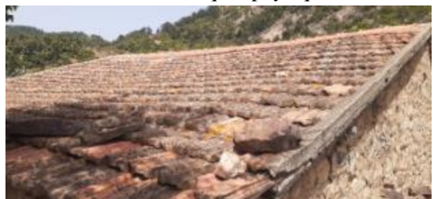
Figure 32: Toiture en tuile village (Boumennsour)
