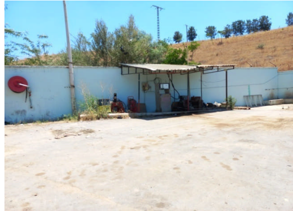
Figure N°11: Station de gasoil
