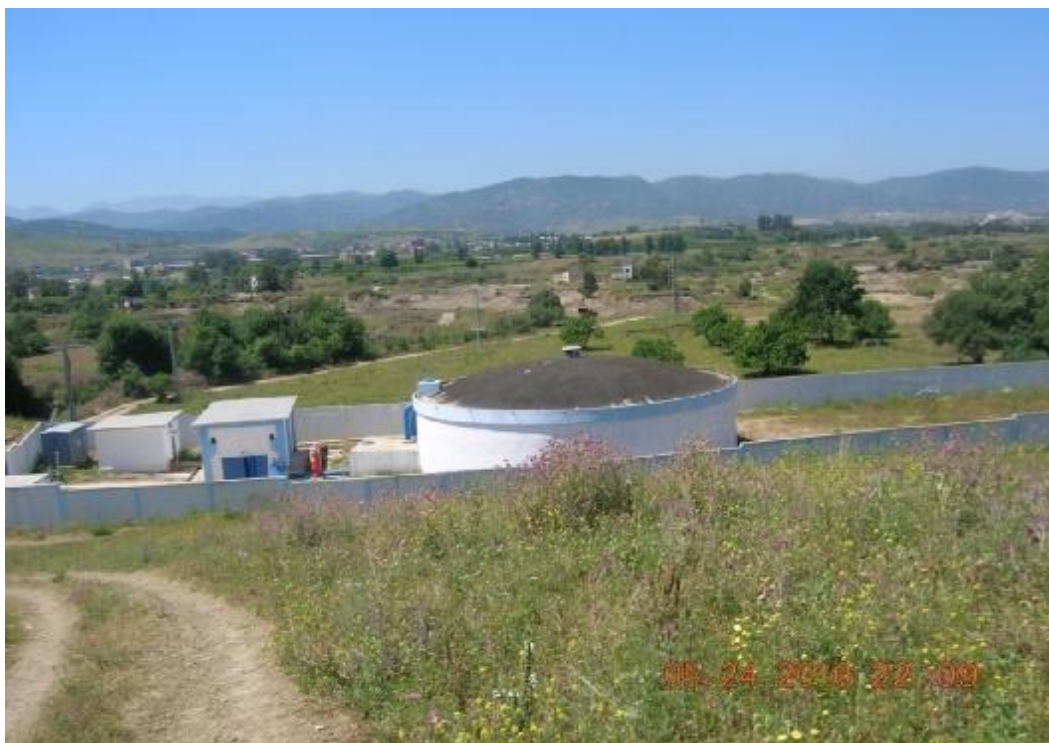
Figure 1.13 : La station de reprise (SR0)
