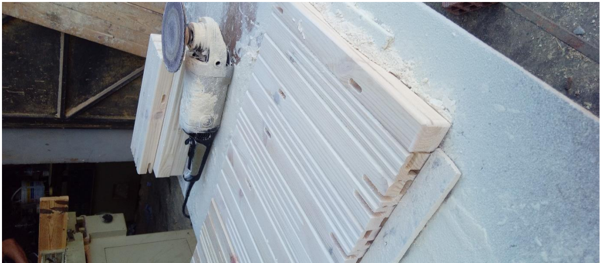
Figure III- 4: Planches en ponçage.
