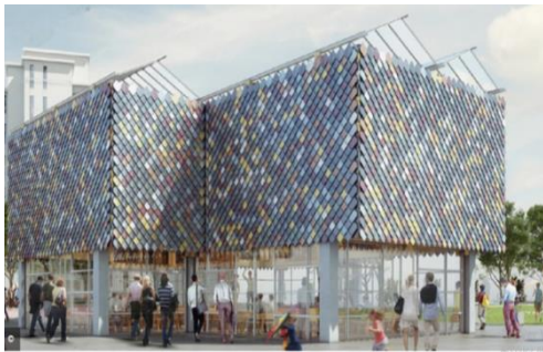
Figure.26: The People's Pavilion. Source: Filip Dujardin, ArchDaily (2019)
