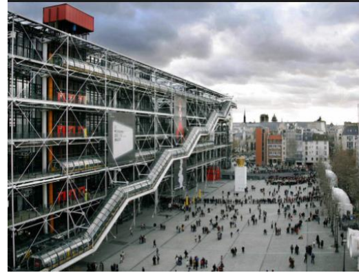
Figure 18 : Centre Pompidou France
