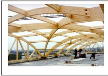
Figure 157: structure lamellée collé
