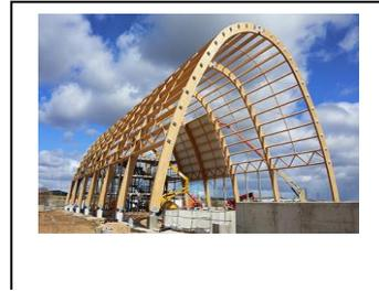
Figure 156: structure lamellée collé
