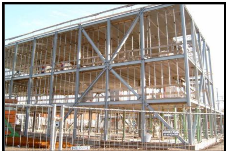
Figure :les contreventement de façades, source :Google
