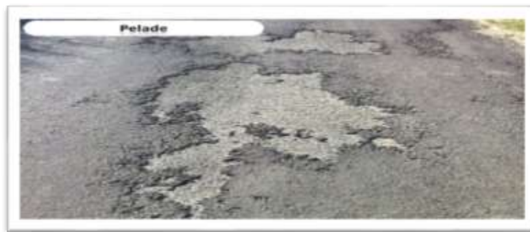
Figure I.20 : pelade (Slideshare, 2013)
