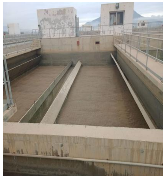
Figure I.4 : Filtres Aquazur V.
