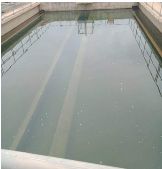
Figure I.4 : Filtres Aquazur V.
