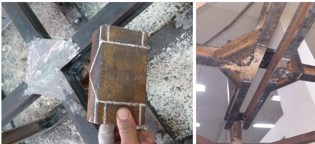
Figure II-29: Éléments de renforts
