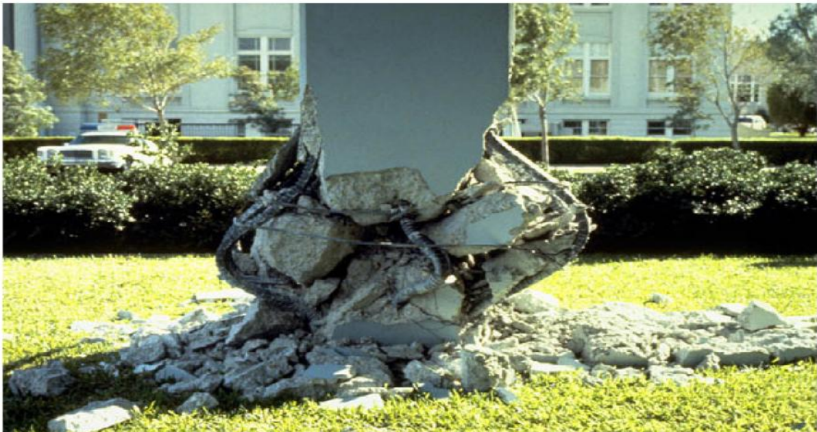
Figure I.11: Non confinement du béton [10]
