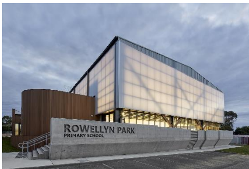
Figure IV 55 exemple d'une double peau en polycarbonate Source : https://danpal.com.au/galleries/rowellyn-park-primary-school/ 17/06/2023
