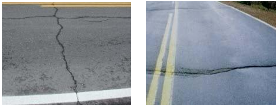
Figure I.19:Fissures transversales.
