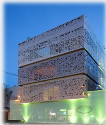
Figure 100: facade du projet.
