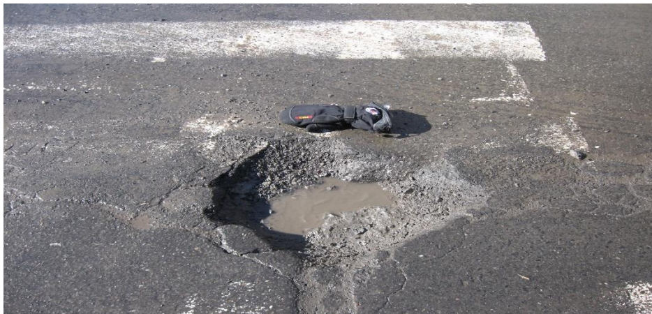
Figure I.21. Nid de poule (Tremblay, 2007)
