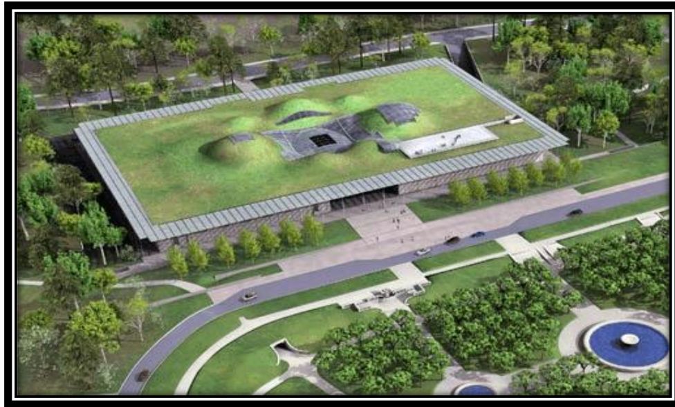
Figure 58: Toit vivant Source: www.calacademy.org
