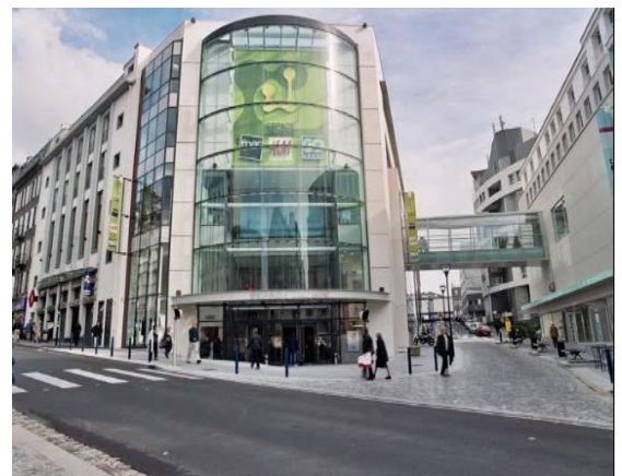
Figure 132: centre commercial de Jaurès
