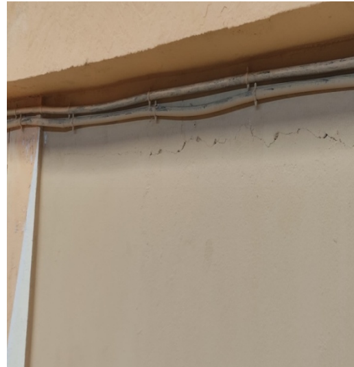
Figure VI.11b : fissure horizontale
