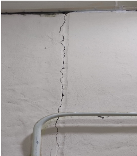
Figure VI.11a : fissure verticale
