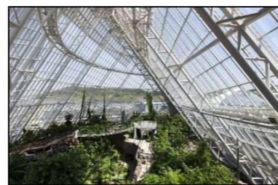
Figure115 : le serre del'ecorium Source : https://www.synchronia.com/en/magazine/
