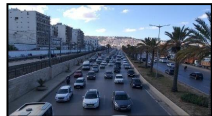
Figure 24: Voie ALN Hamma.
