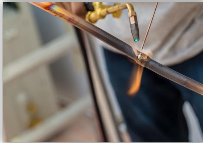
Figure II.41 : Le soudo-brasage
