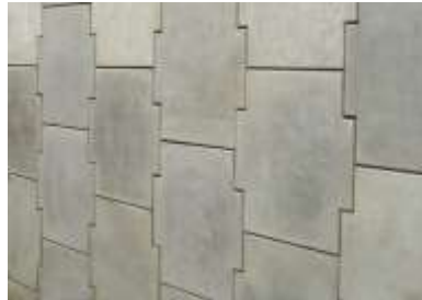
Figure 1. 11:: Ecailles cruciformes
