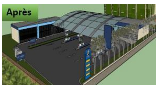
Figure 56 la station multiservice.
