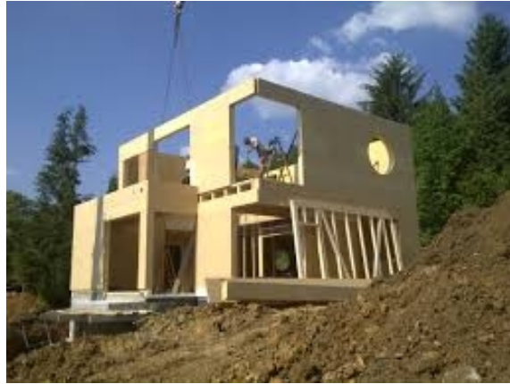
Figure 12 : Construction aux terrains de forte pente[1]
