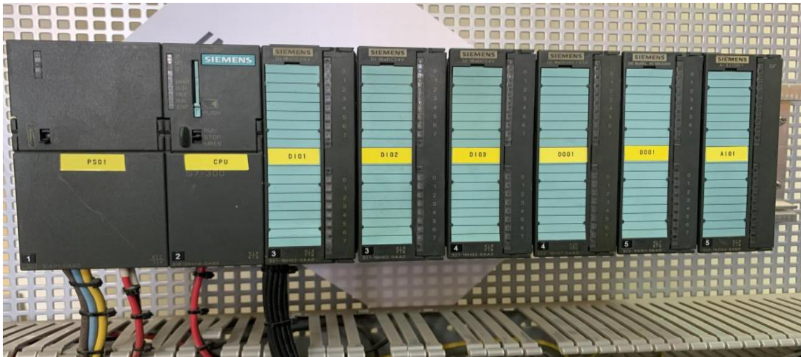
Figure III.8 : Automate S7 300.
