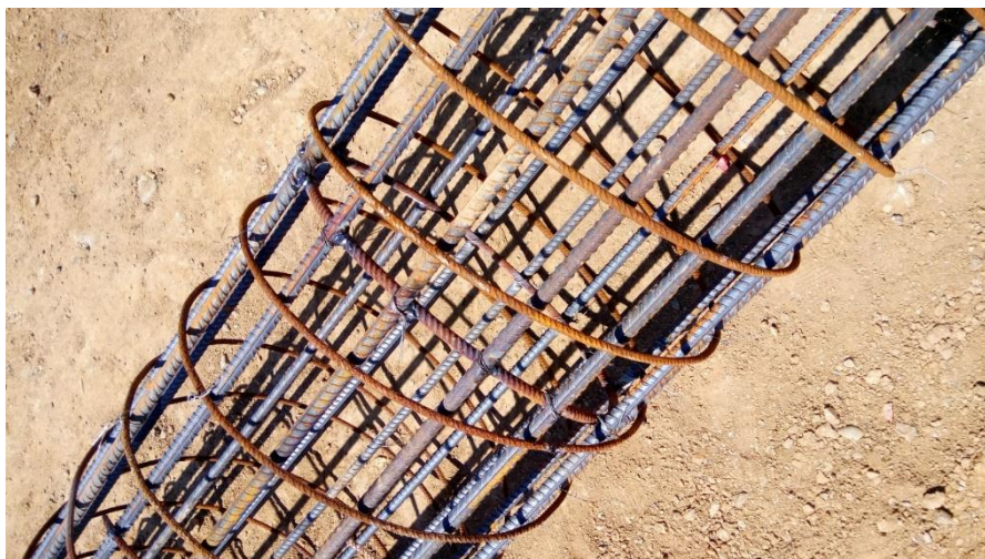
Figure I-22 confinement spirale [38]
