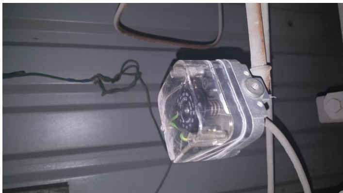
Figure 1.9.2 pressostat de pression
