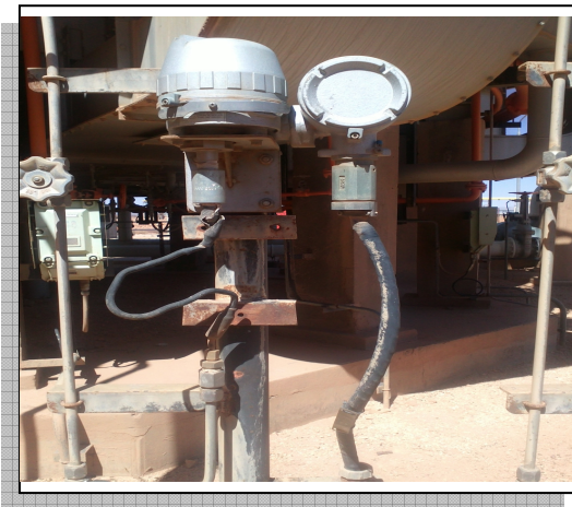
Fig II.6: Pressostat
