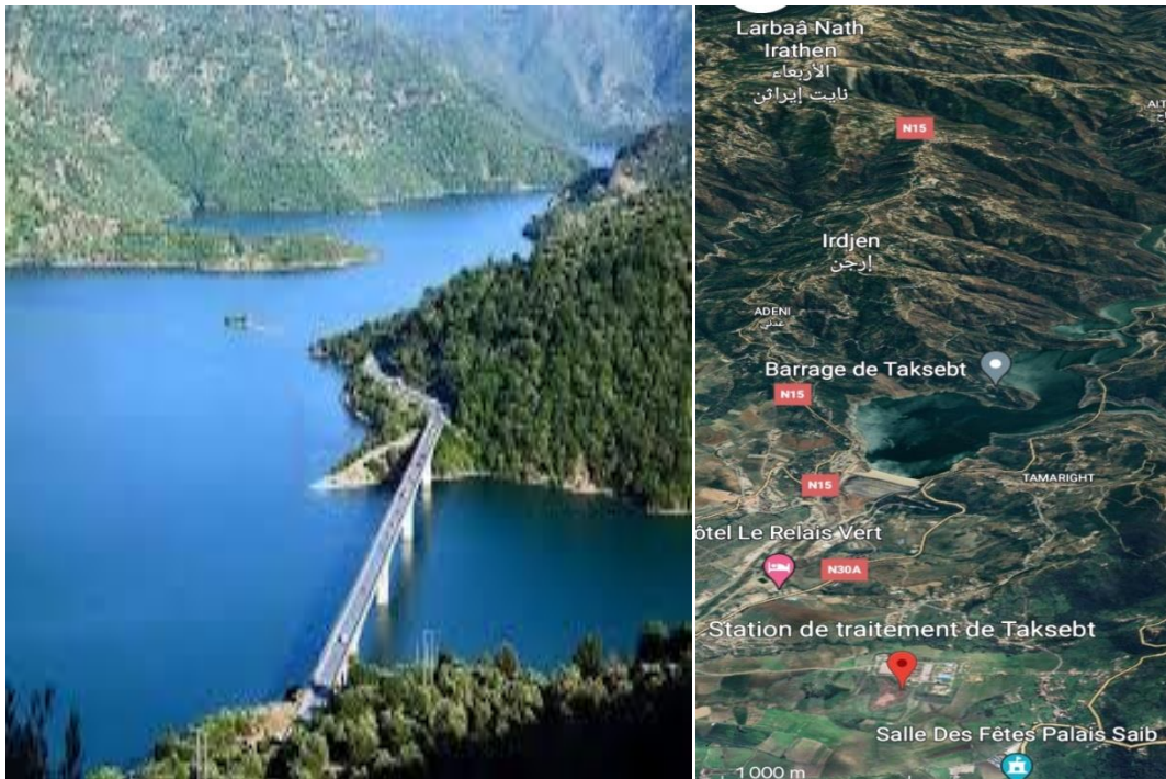
Fig.4: barrage Takesabt Tizi-Ouzou(Google earth.2024)
