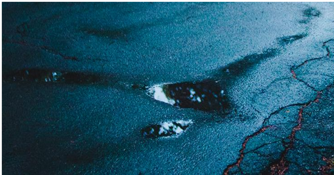
Figure I.10. Les flaches (McClean, 2020).
