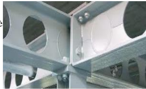
Figure 97 : assemblage poteau-poutres Source : google image
