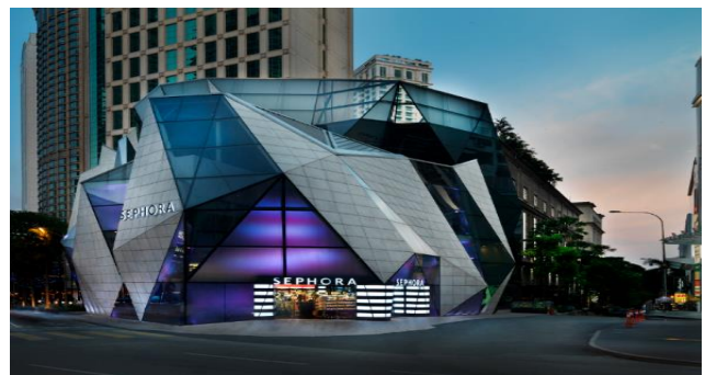
FIGURE 97: STARHILL GALLERY APRES LA RENOVATION EN 2011.
