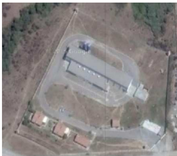
Figure I.4 : la station de pompage[14]
