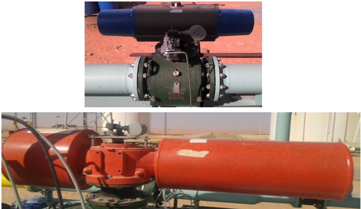
Figure 3.18 : La vanne SDV
