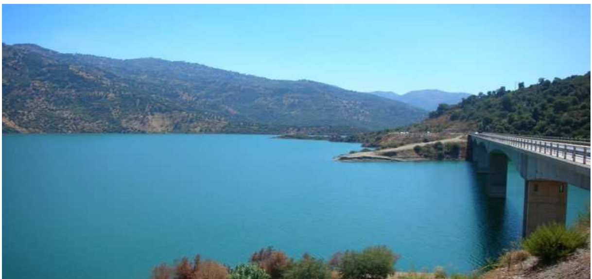
Figure I.1 Barrage de Taksebt
