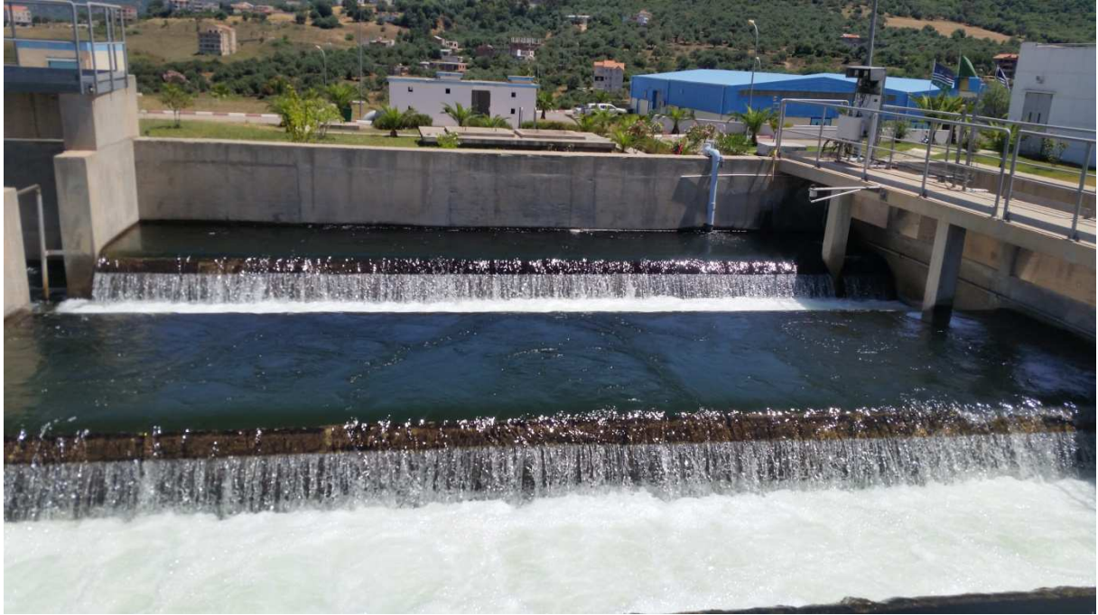
Figure I.6 Chambre de dissipation.
