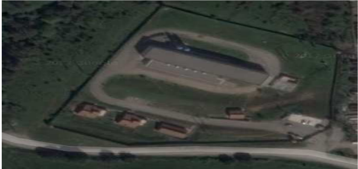
Figure I.2 : Station de pompage.
