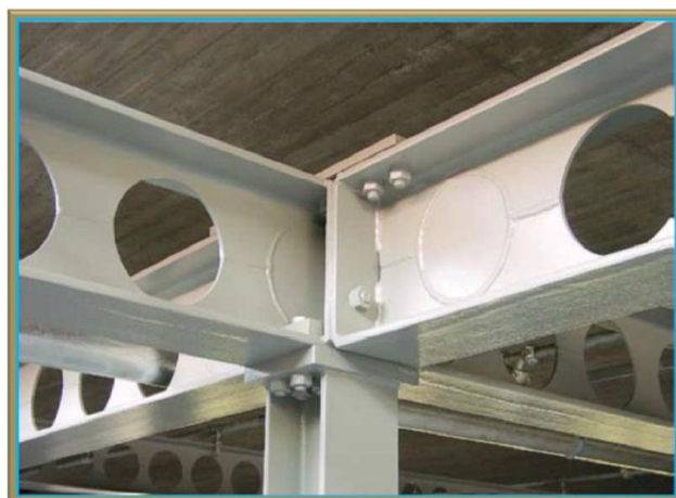
Assemblage poteaux-poutres
