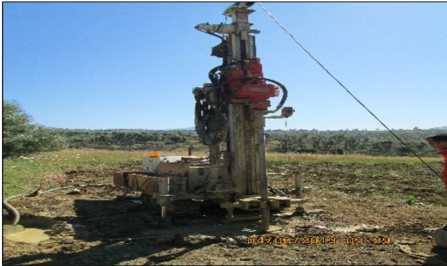
Figure III.3:Essais in situ (Sondage carotte)
