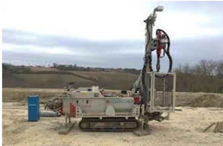
Figure III.4: Essai in situ (Essai pressiométrique)
