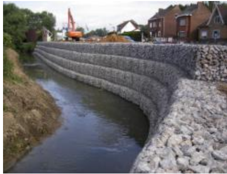
Figure (I.15) : Le gabion.
