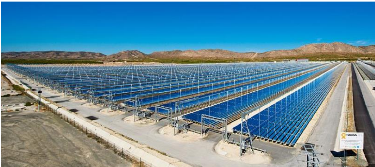
Figure 26: centrale solaire a miroir Fresnel
