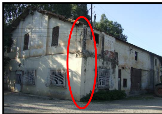
Photo 4.92: fissure verticale
