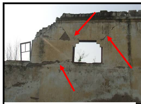
Photo 4.102: Fissures diagonales
