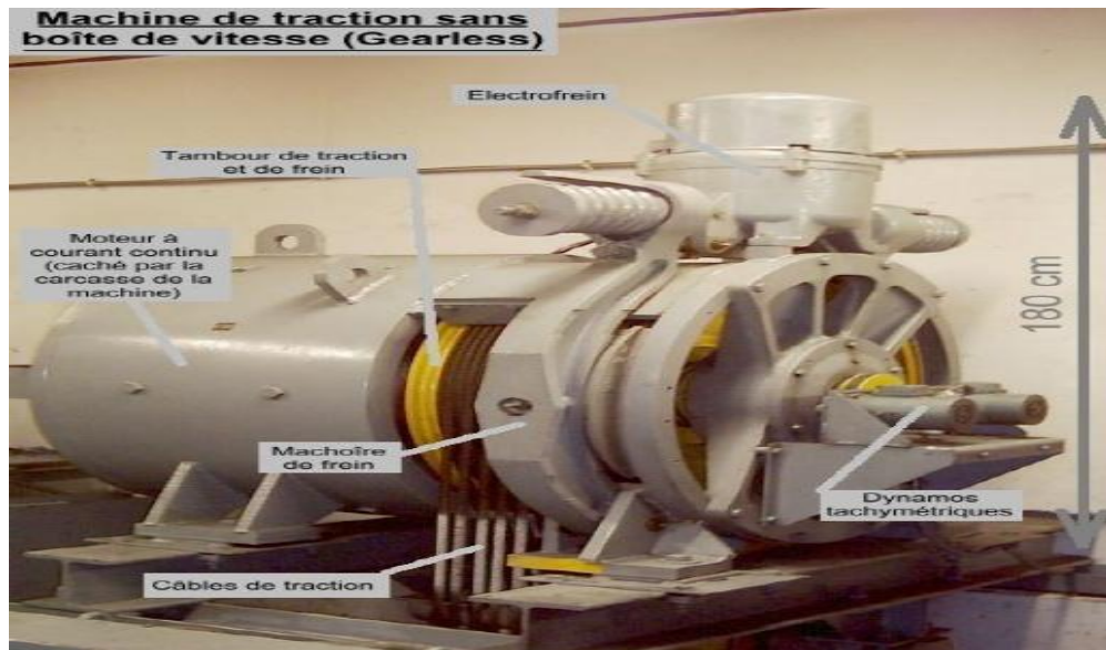
Figure I.13: Machine de traction "Gearless".
