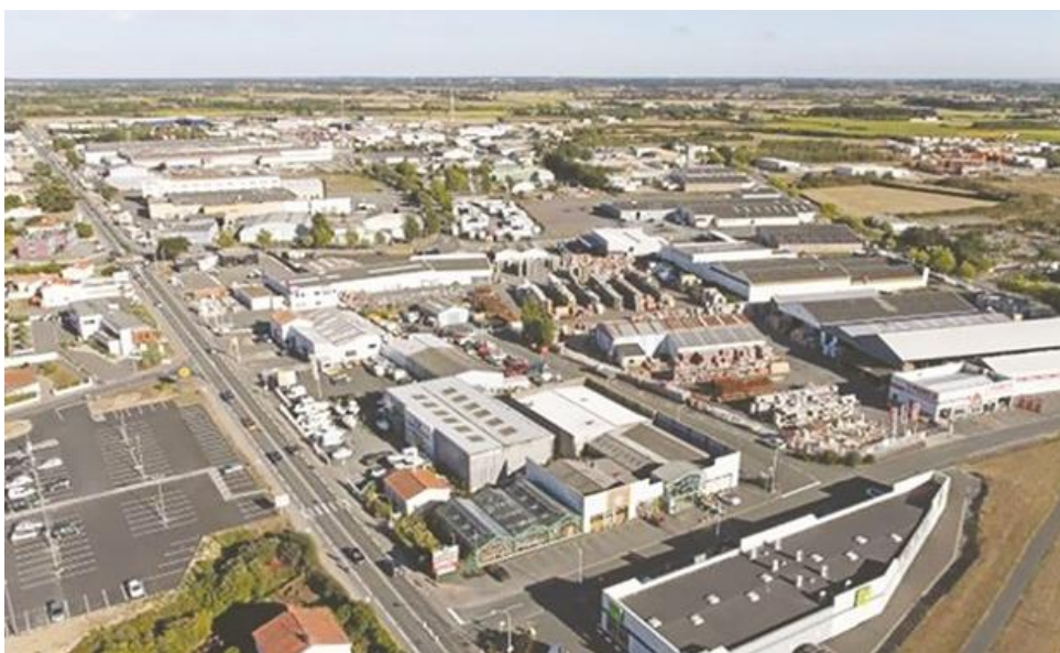
Figure 9 Zone industrielle de Reghaia
