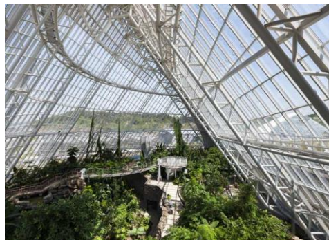
Figure 35: structure supportant le vitrage
