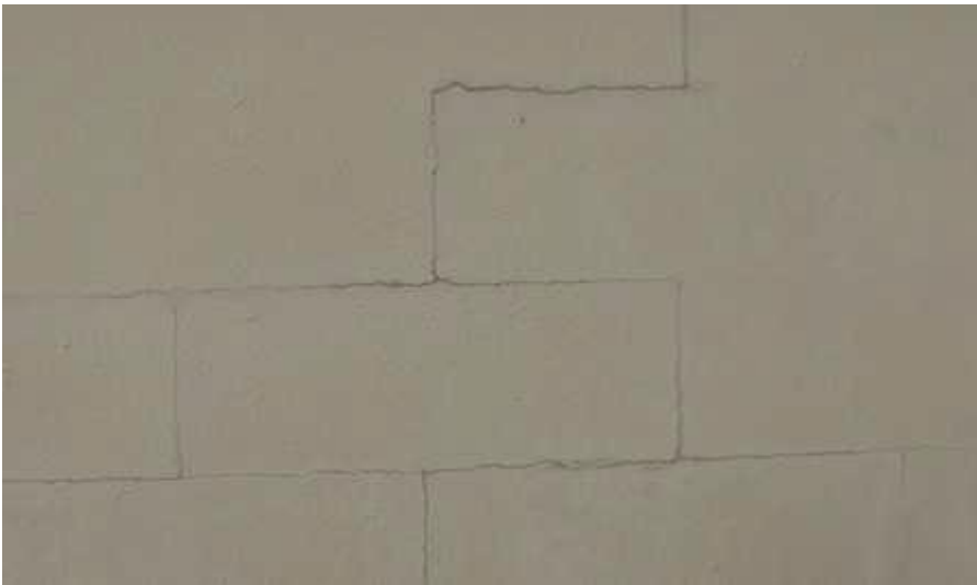
Figure II.1 : Microfissures
